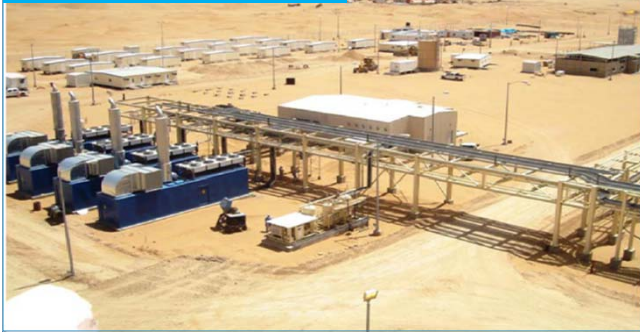
Accommodation & Life Support Area.
