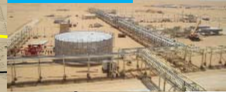
Hot Area Processing Train
