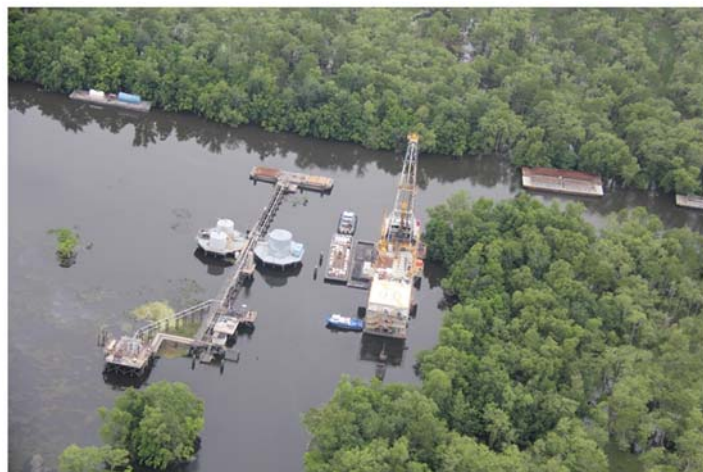
Williams No.2 discovery well: Barge drill rig next to production & oil storage facilities
